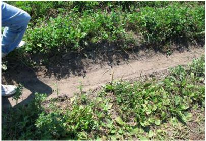
Photo 409, Point4: Rutting on Levee Crest.
